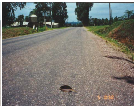
D425 Alverston – Waterproof Gravel 8 months after construction
