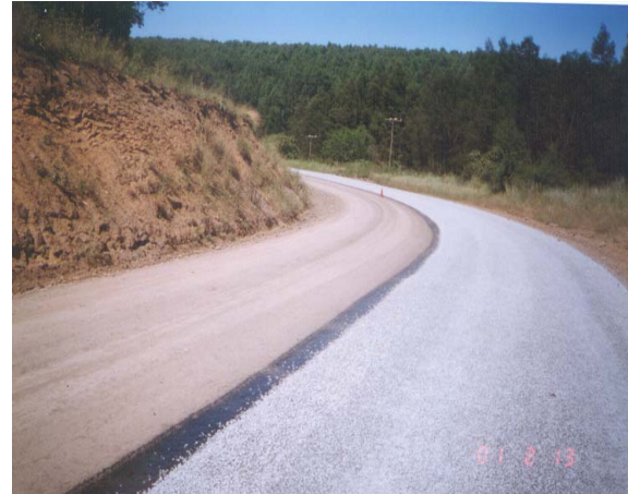
P 16/2 Kranskop - Application of half the cutback 150/200 penetration grade Bitumen binder and the graded aggregate for the Gravseal. Note the exposed binder for the center joint overlap.
