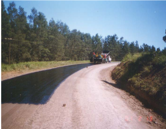
P 16/2 Kranskop - Application of the cutback 150/200 penetration grade Bitumen binder for the Gravseal on the lime stabilised base layer.
