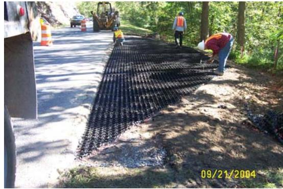
b. Ring and grid installed and cut to shape.
