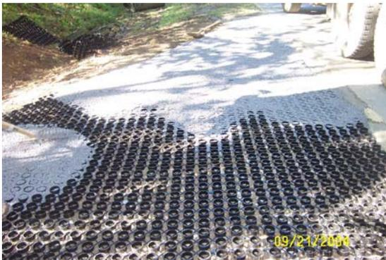
c. Backfill consisting of AASHTO #89 stone.
