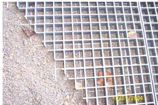
b. Grate placed on weld wire fabric and #89 stone.
