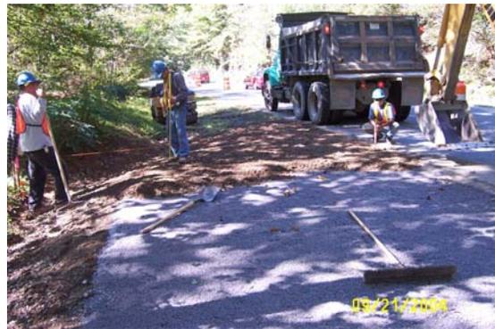
d. Aggregate-topsoil cover for turf establishment.
