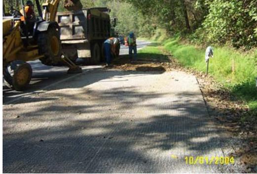
c. Aggregate-topsoil covering grating system.
