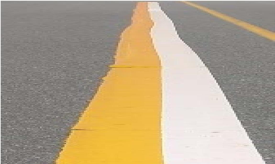
FIGURE 2. CENTERLINE POLYESTER MARKING MATERIAL ON ASPHALT WITH TYPE I BEADS
