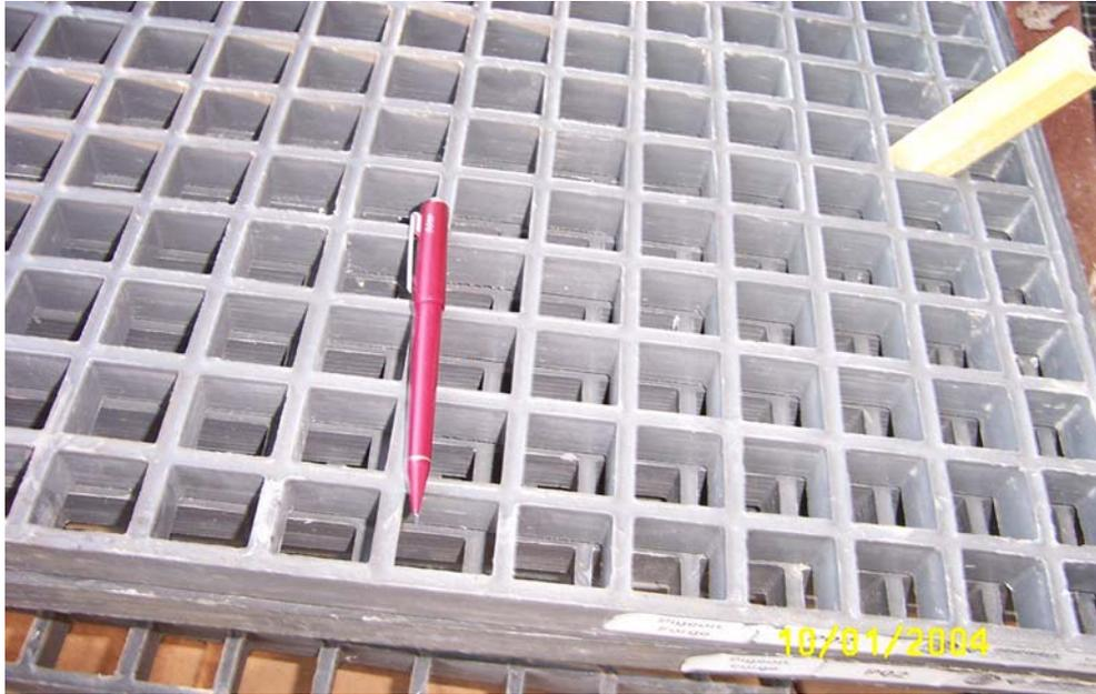
Figure 7. The fiberglass grates for this project were one-inch deep and were delivered in 4' x 10' sheets. The panels for this project were pre-cut to the shape of the parking areas.
