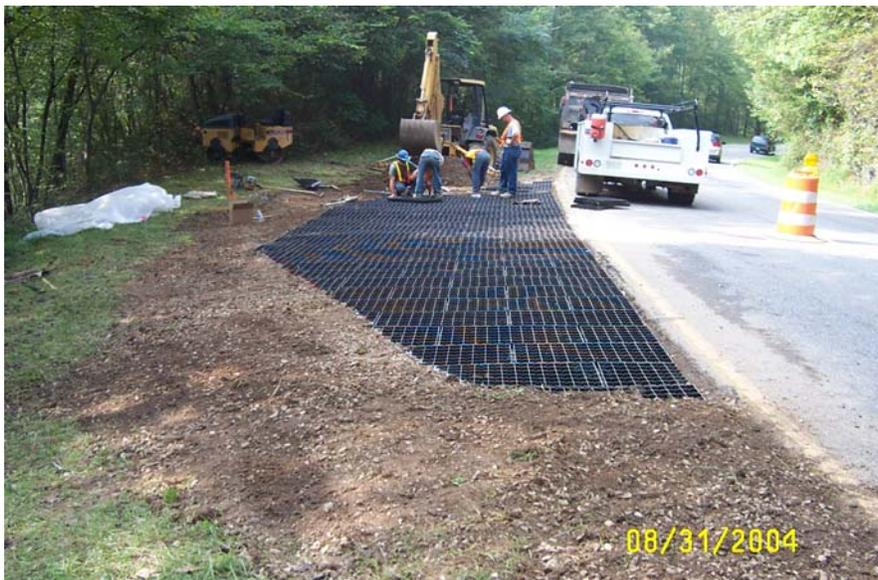
Figure 4. Geoblock installed and cut to fit the pull-off at PA #3.
