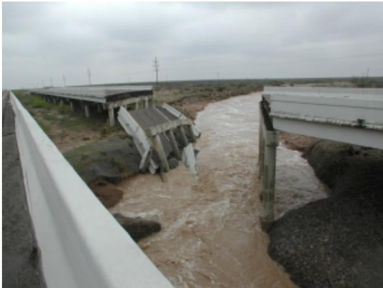
A bridge along Interstate 20 just east-northeast of Toyah over the normally dry Salt Draw failed Sunday evening. This failure was the result of fast-moving flood waters originating from previous heavy rainfall over the Davis Mountains. Hydrologists also credited a residual flow of water through the draw from the Toyah dike break early Sunday for contributing to the gradual process that caused
