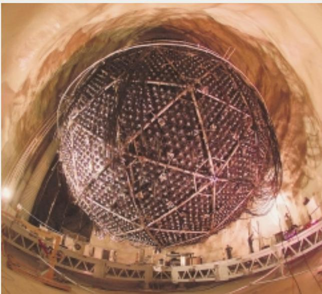
**Counting nature’s phantoms.** The SNO neutrino detector, shown here before it was filled with water, is located 2000 m underground at the Creighton mine in Canada. The geodesic structure that supports the detector’s 9500 photomultiplier tubes is shown inside the rock cavity excavated for the detector. The complete detector contains 7000 tons of ultrapure water, surrounding a 12-m-diameter transparent acrylic sphere filled with 1000 tons of ultrapure heavy water.
